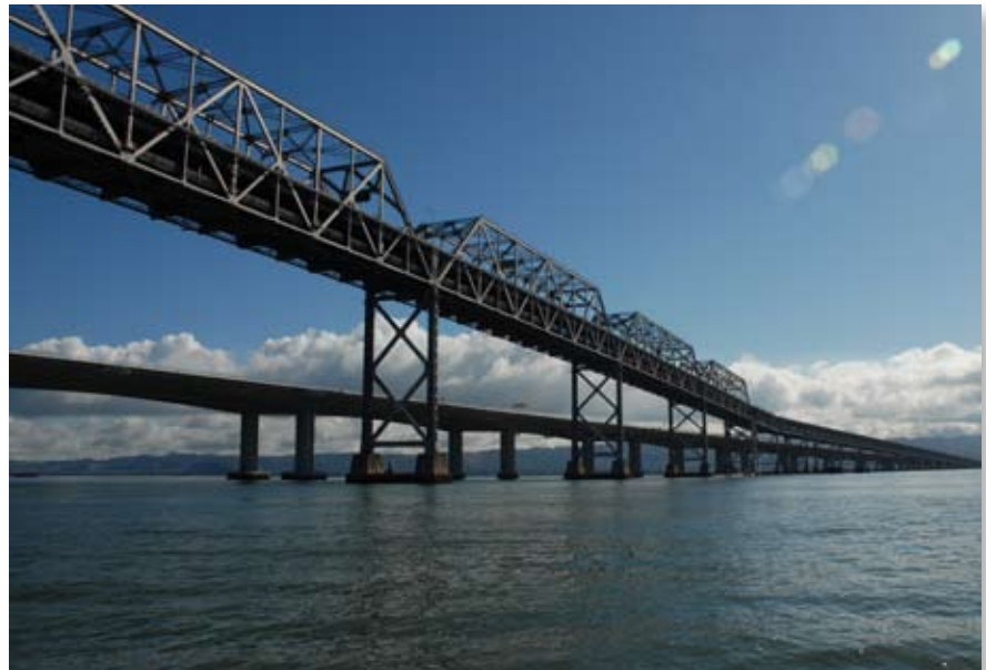
On the way to Petaluma—Bay Bridge old and new.
